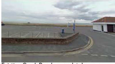
Existing Creek Road car park takes up a prominent position of the site overlooking the beach and seafront.
