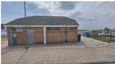
Unattractive and dated public toilets
