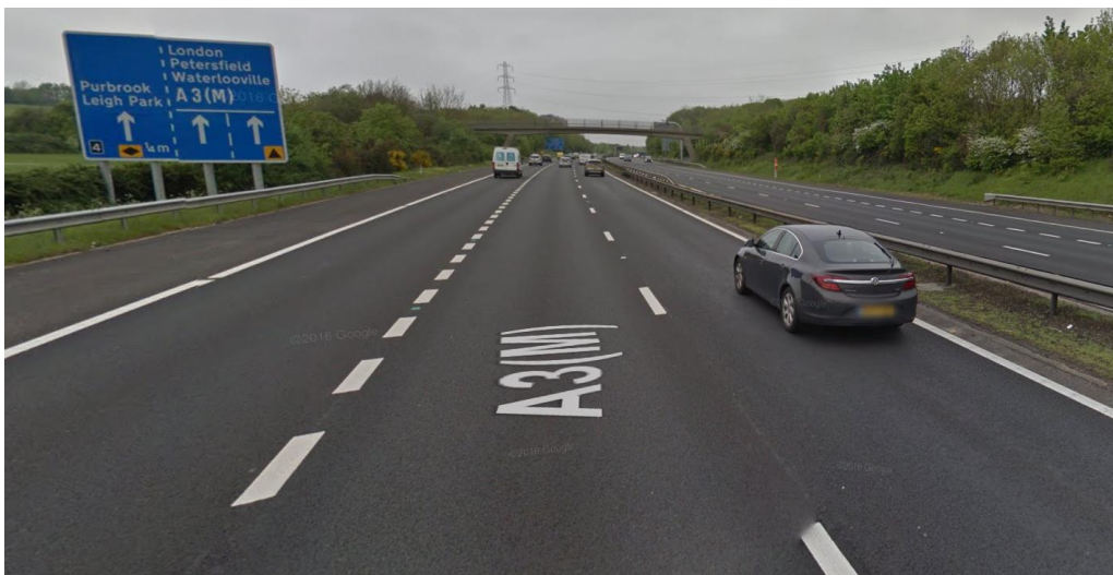
Example of lane gain / lane drop between J4 and J5 of the A3M (credit: Google)
