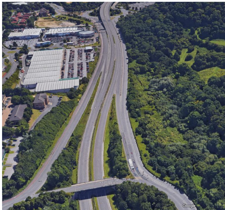
Example of parallel link roads on the A38 in Plymouth. Traffic from the previous junction (nearest the camera) merges with the off-slip from the A38 mainline (centre) and to access the A38 proper must pass through the succeeding junction furthest from camera (credit: Google ©). This would be the arrangement adopted for eastbound traffic from Warblington in option 4A above, having to pass through the new Southleigh junction to access the A27 mainline. Note however how close the slip road can be placed to the main carriageway.
