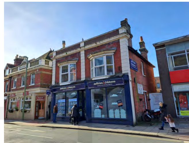
The replacement of the original timber windows with uPVC units on the first floor depreciates the contribution of this historic building to the streetscape.
