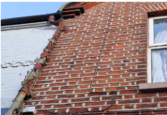
The primary façade of this building been repaired using ribbon pointing, where mortar is applied in thick, raised bands. This affects the ability of the brickwork to expel moisture and causes issues with staining and algal growth. It can ultimately lead to the brick crumbling away.
