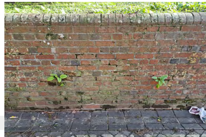
Vegetation growth and missing pointing to a section of the boundary wall with the churchyard on Homewell. A plant will typically root in mortar joints and force itself deeper as it grows, which can push the built fabric out of position and weaken the integrity of the wall.
