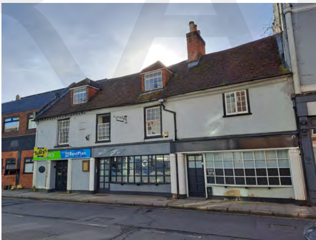
This terrace of shops on East Street is suffering from failing render and exposed/rotting woodwork.
