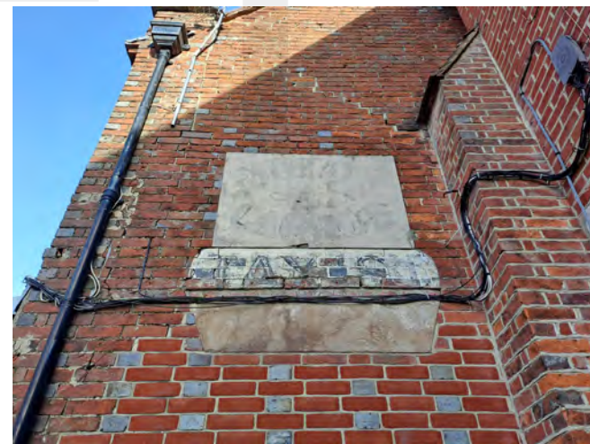
Trailing wires distract from the historic and aesthetic interest of this side elevation on South Street, which evidences multiple phases of brickwork and two ghost signs.
