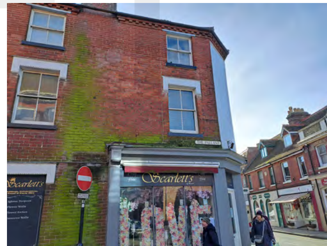
Heavy algal growth to a section of brick wall on The Pallant indicates water run off is not being managed effectively.
