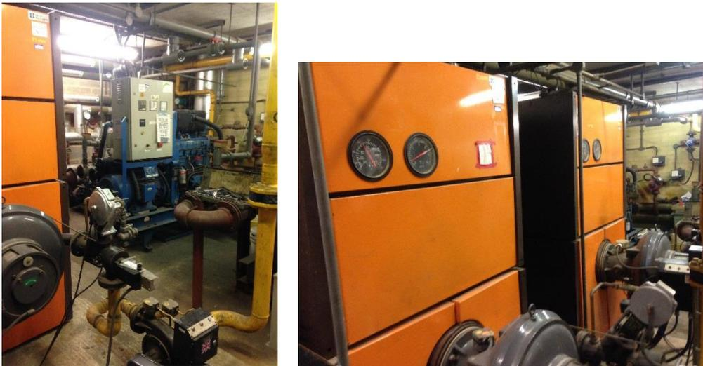
Figure 5.1 Existing CHP and gas boiler plant within 'wet-side' leisure centre plant room
