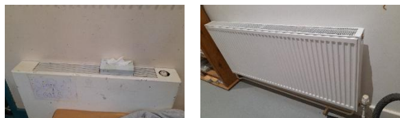
Examples of existing radiators with TRVs.
