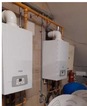
Existing gas boilers (left) and gas water cylinder (right) at Acorn Centre.
