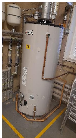
Existing gas boilers (left) and gas water cylinder (right) at Acorn Centre.
