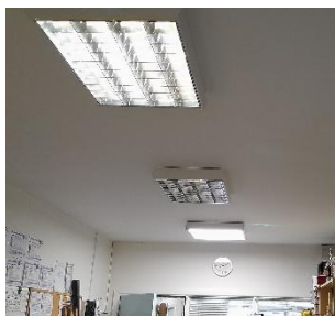
Examples of existing fluorescent fittings in Acorn Centre.
