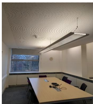
Existing linear fluorescent fittings in open plan offices (top) and meeting rooms (bottom).
