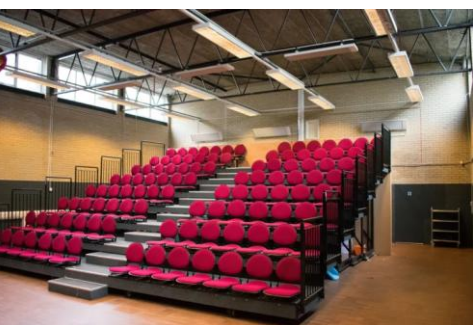
Example of electric IR heaters in high ceiling venues.
