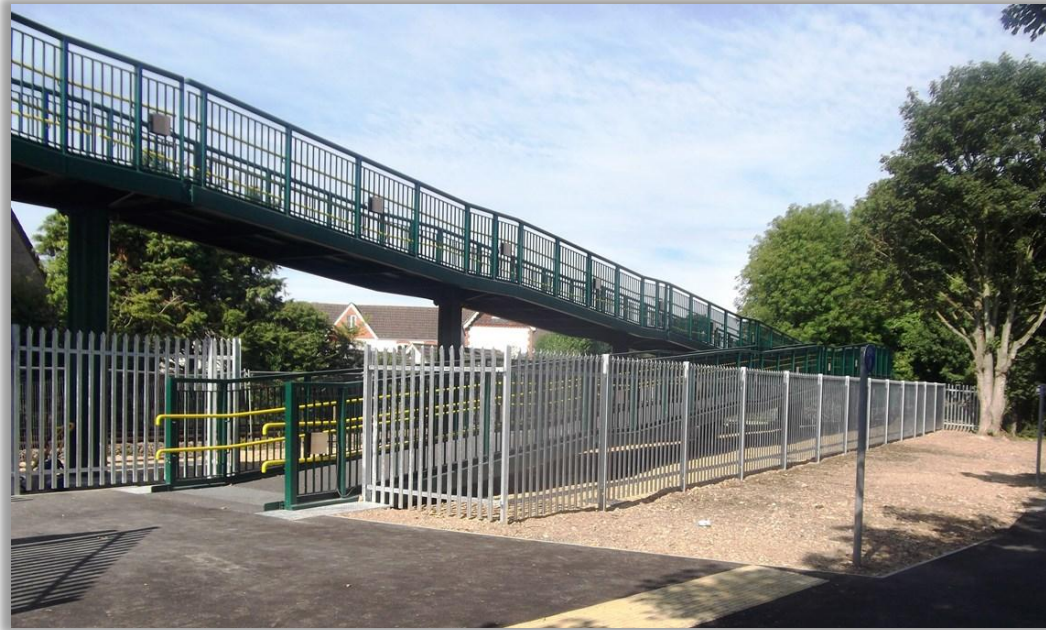
Figure 2B – steel folded span and approaches at Fishbourne, West Sussex © Network Rail
