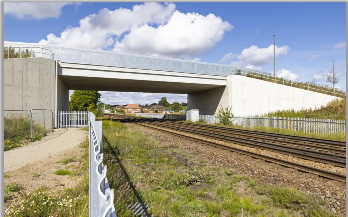
Figure 5B – Stonehill Road bridge, Ash © Volker Fitzpatrick
