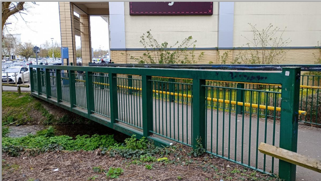
Figure 1 –Solent Retail Park bridge as example of Vierendeel girder span
