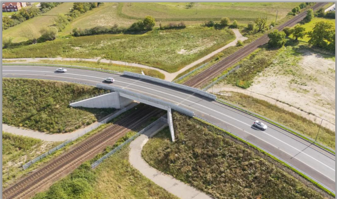
Figure 5A – Stonehill Road bridge, Ash © Volker Fitzpatrick
