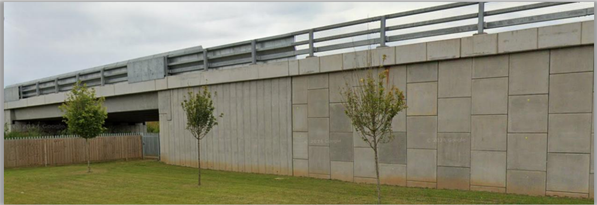
Figure 4 – Lyminster bypass, Littlehampton showing crib wall solution for approach embankment, with minimal land take © Google
