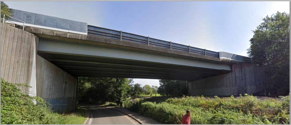
Figure 3 – Long Road overbridge, Petersfield, showing a typical composite structure © Google
