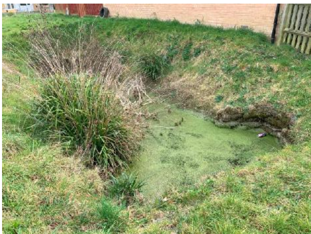
Photograph 4.12: Balancing Pond P1 connected to Ditch D1 via a culvert, east of the Site boundary
