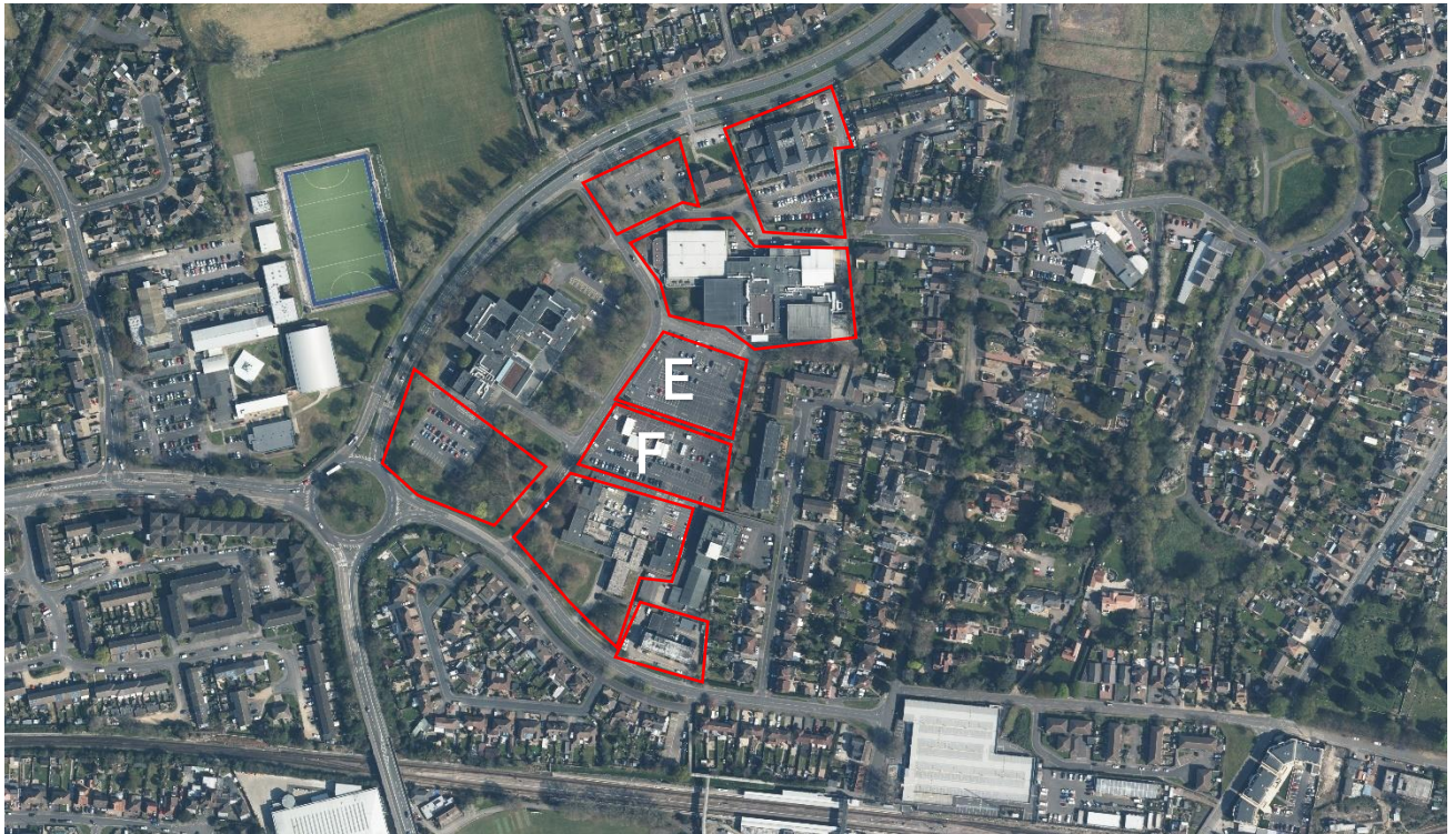
Aerial photograph showing the Havant Plaza sites E & F outlined in red
