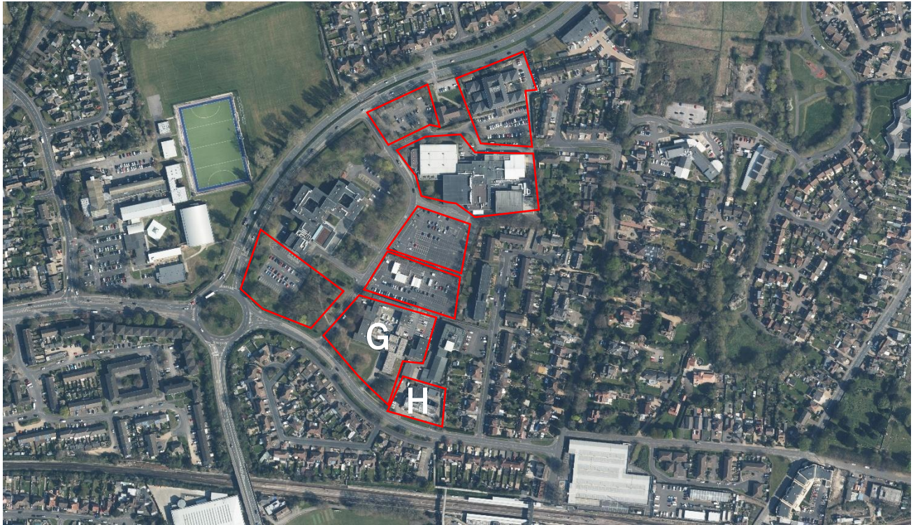
Aerial photograph showing the Havant Plaza sites G & H outlined in red
