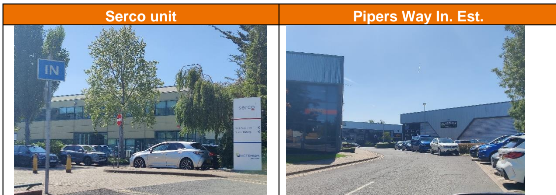
Figure 5-13 Examples of industrial units, Brambles Business Park/Elletra Avenue
