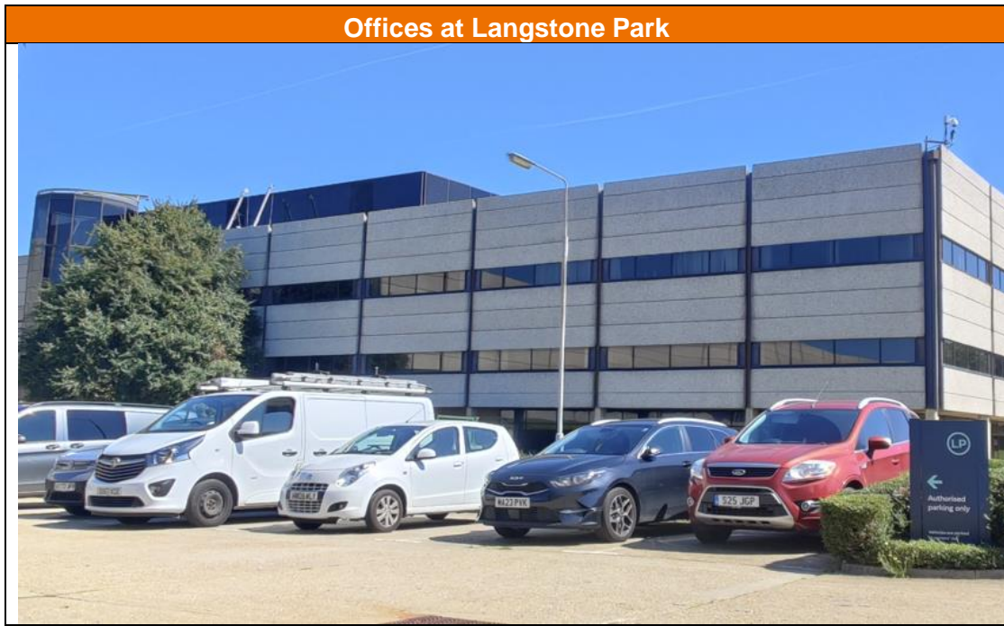
Figure 8-2 Examples of offices at Langstone Park
