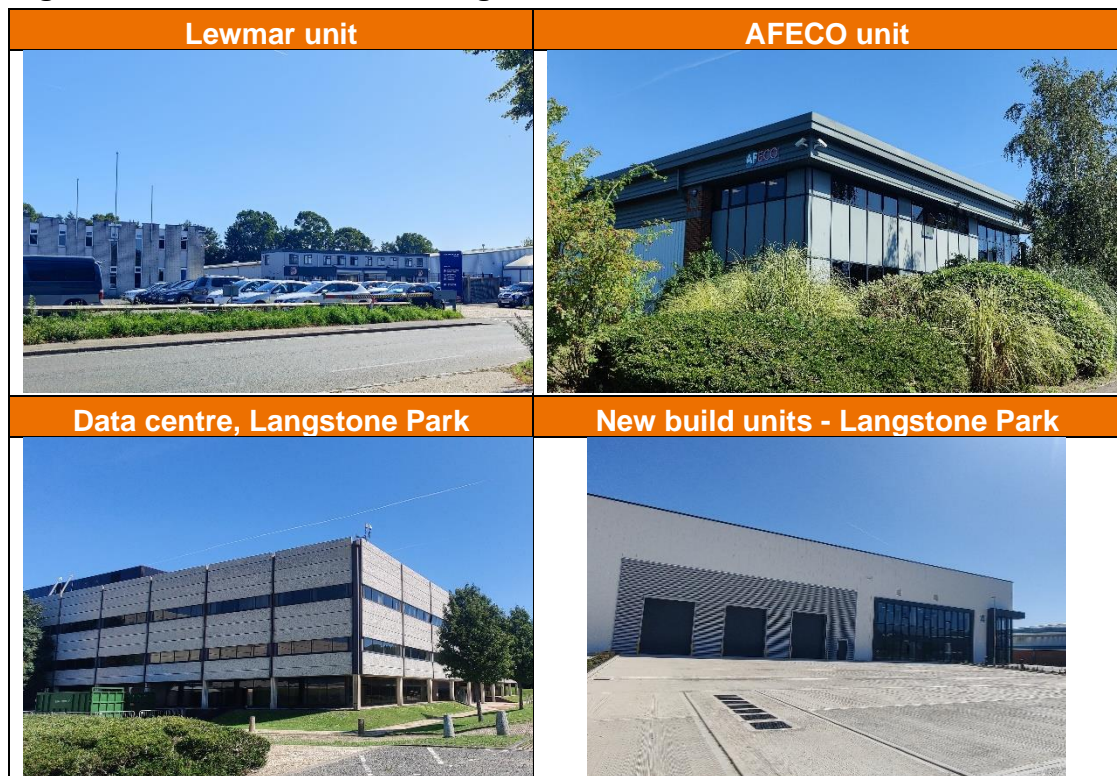
Figure 5-8 Industrial units, Langstone Park/ Southmoor Lane
