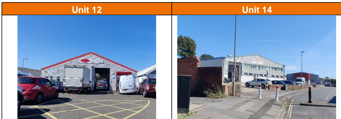
Figure 5-5 Examples of industrial units, Tanneries
