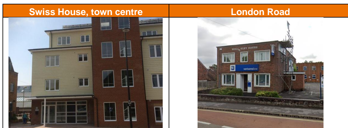
Figure 8-3 Examples of offices at Waterlooville Town Centre/London Road
