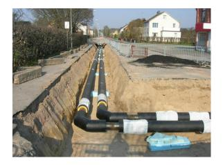
Figure 6.4 Image of typical pre-insulated heat pipe
