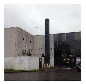
Figure 5.8 Proposed location for biomass storage outside existing 'dryside' plant room. Existing chimney could be used to house biomass flue, subject to structural survey.
