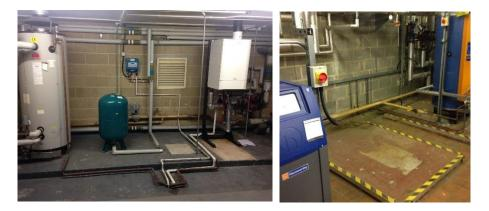
Figure 5.10 Space available to accommodate new plate heat exchanger to connect to district heat network (Havant College Sports Hall Plant Room, Havant Health Centre)
