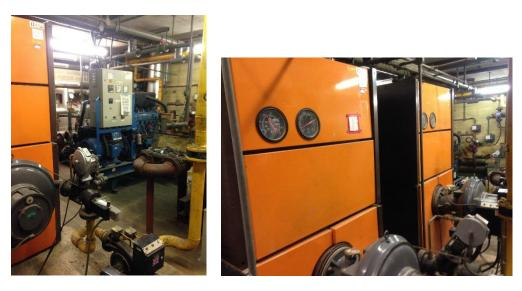
Figure 5.1 Existing CHP and gas boiler plant within 'wet-side' leisure centre plant room
