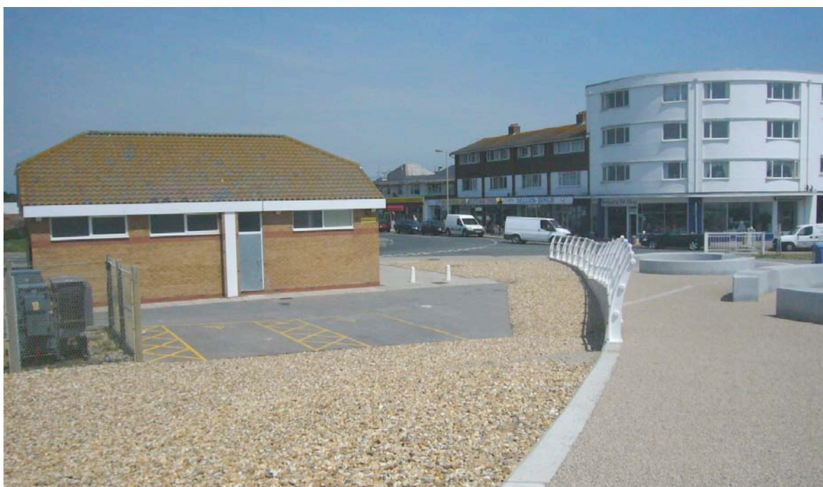
Site for bandstand adjacent to the public toilets
