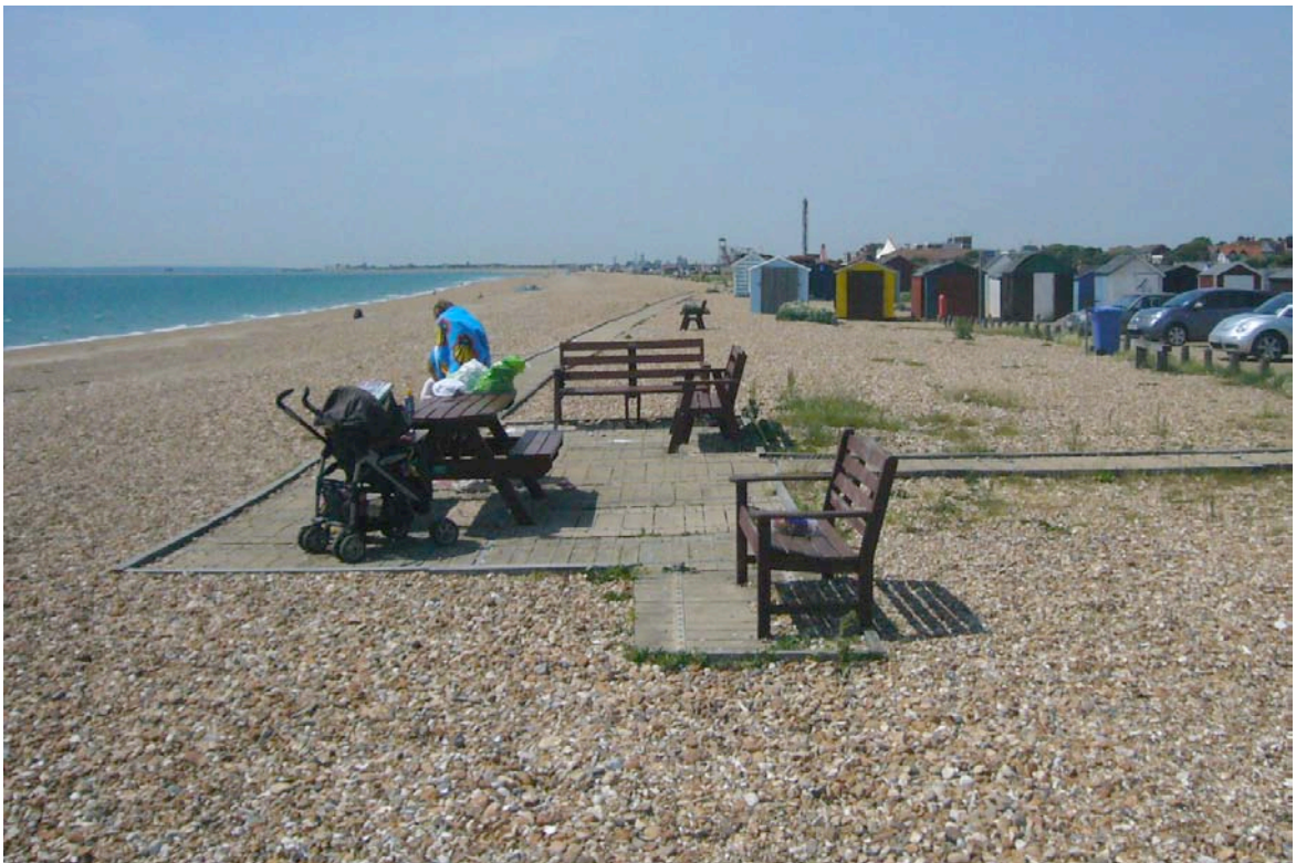
Existing boardwalk by car park – end of Section B
