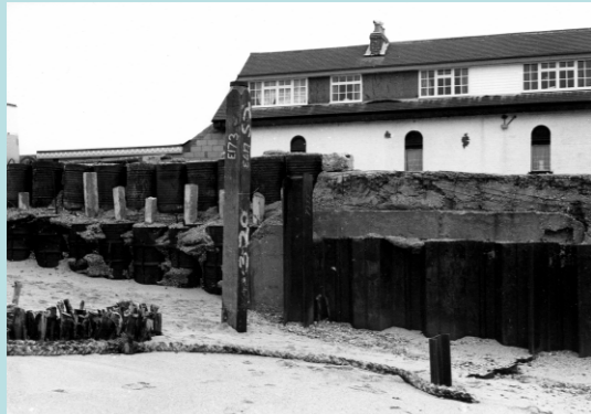
Start of construction, Dec '75
