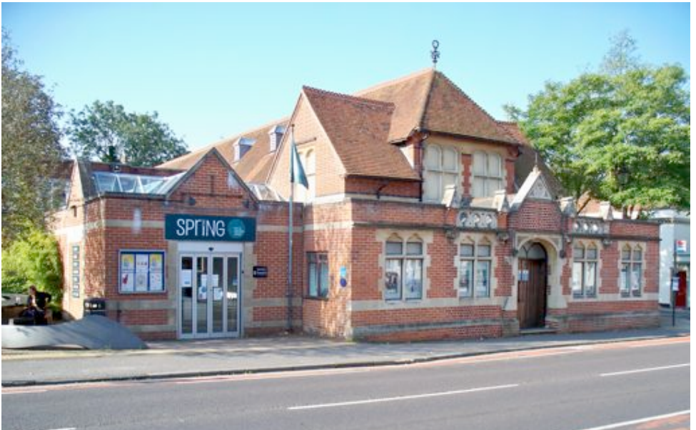
The Town Hall is now the Arts section of The Spring.
