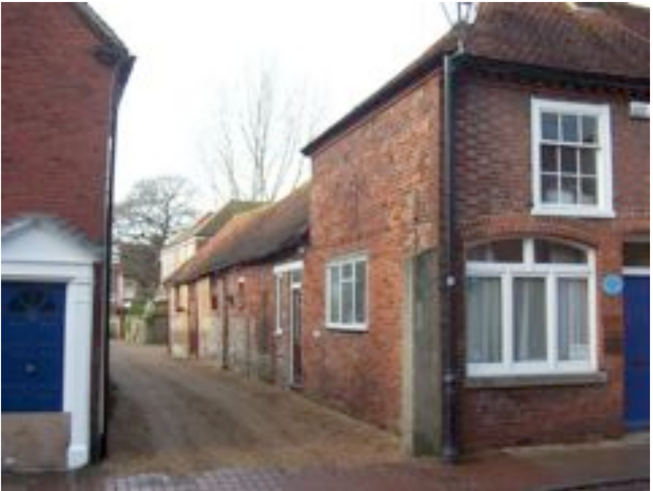
Entrance to the former Jolliffe Malthouse and Brewhouse, South Street at the present day.
