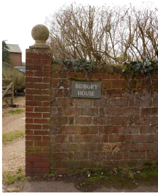
Figure 18: Wall in rat trap bond to Bidbury House
