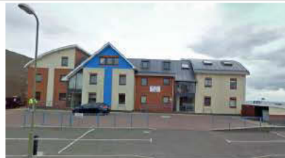
Existing new buildings are poorly designed
