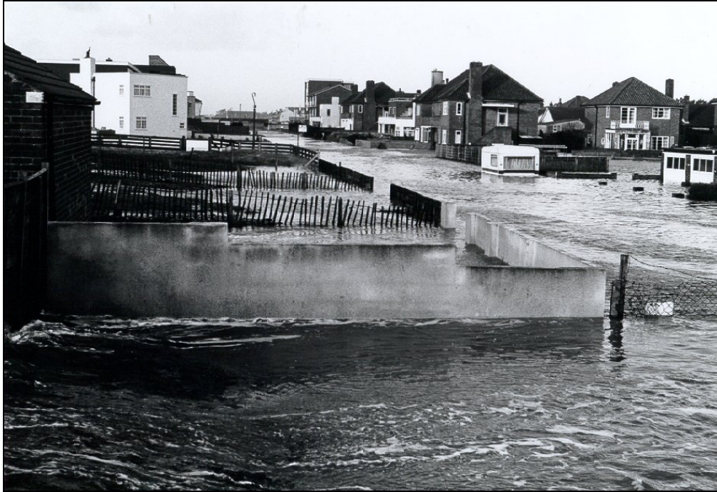
Photo 1 Overtopping flooding at Bembridge Drive 1978
