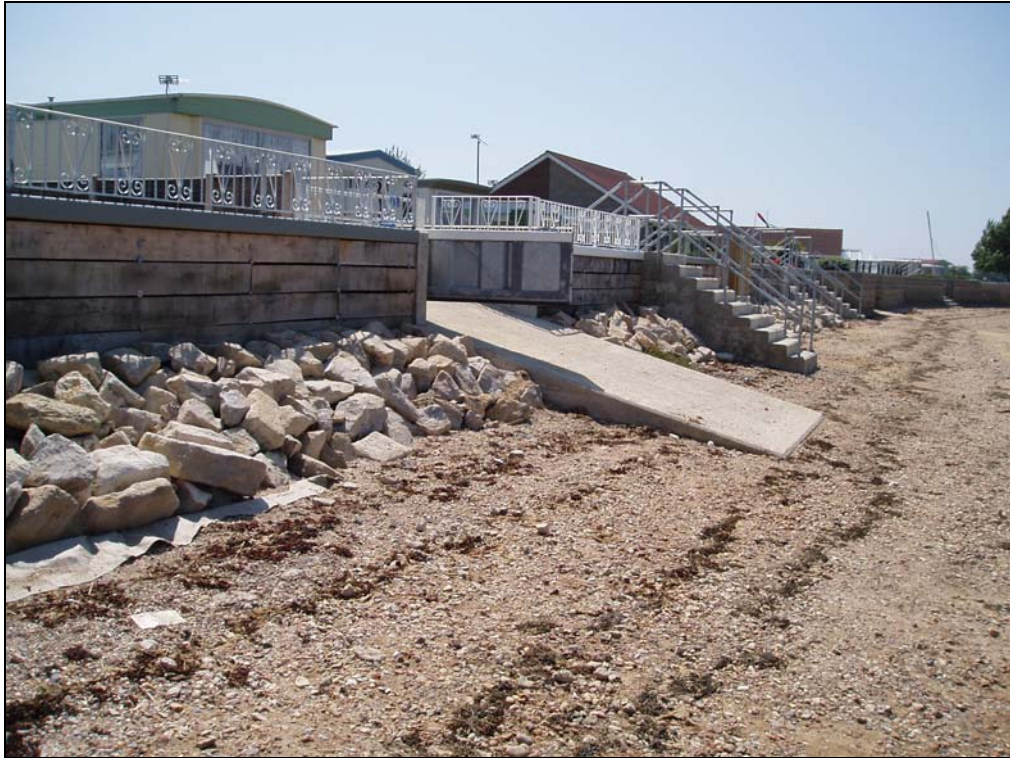
Photo 20: New rock revetment and slipway along southern frontage (12/07/05)
