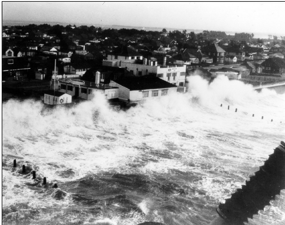
Photo 2 Pre-1985 Wave overtopping seawall at Creek Road/Beach Club
