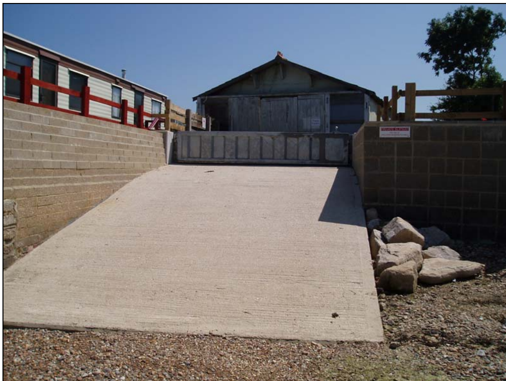
Photo 22: New floodgate and slipway (12/07/05)
