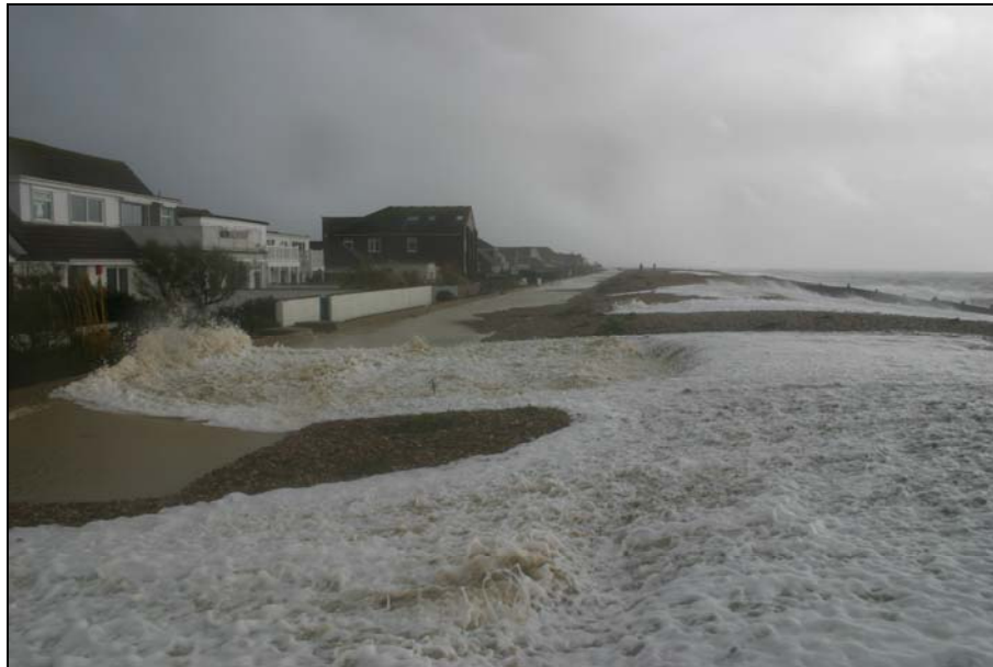
Photo 3: Overtopping wave (view east)
