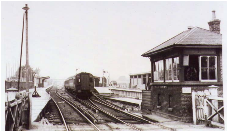
New direct line electric 'Nelson Stock' passing through the new station under construction in 1937. The Havant West signal box and North Street level crossing were still in operation.
